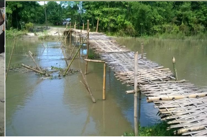
Bamboo bridge to access the village.
